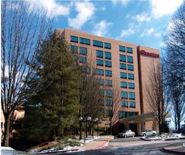
Front of the Building - West Elevation
