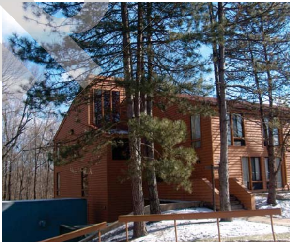
Side of the Building - North Elevation
