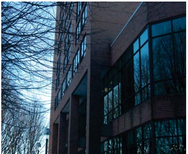
Rear of the Building - East Elevation
